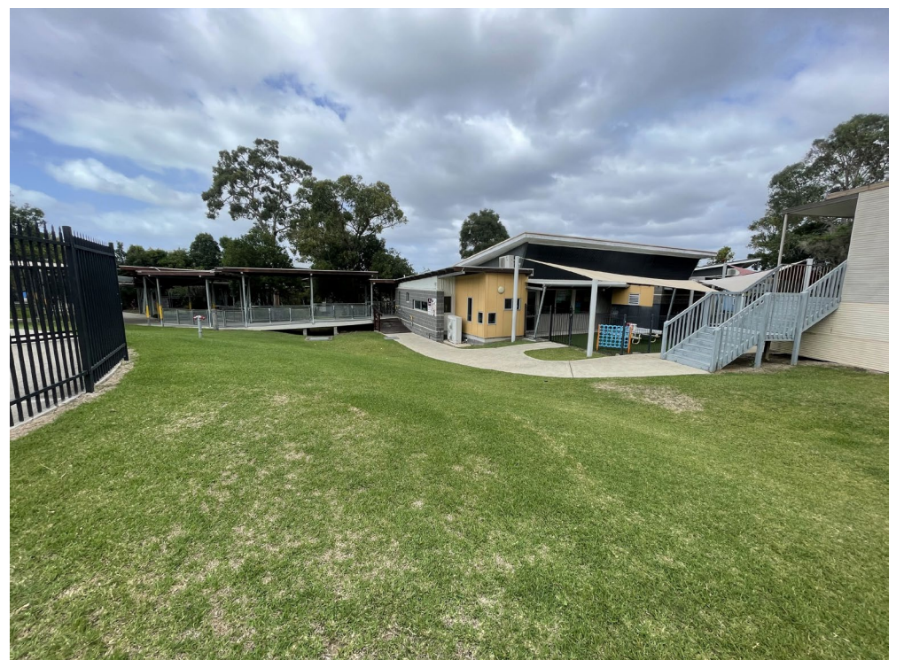
Photo 10: Overview of the northeastern portion of the investigation area adjacent to the school's external fence line. Looking south.
