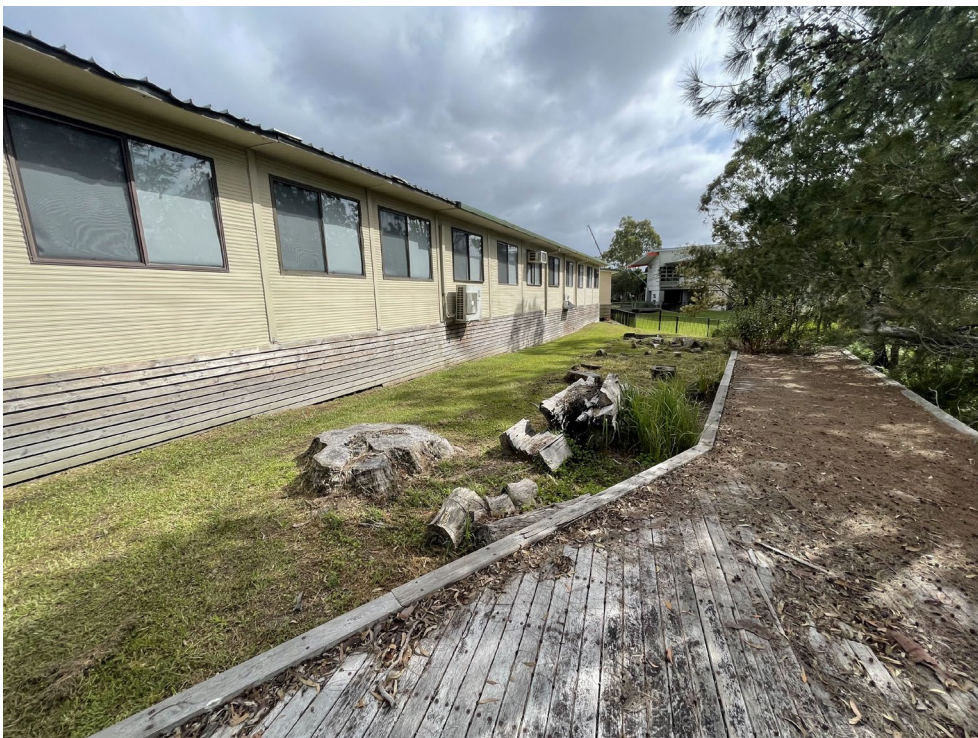
Photo 9: Overview of the southeastern portion of the investigation area showing the old weathered wooden boardwalk present and the rear portion of the primary school buildings present here.
