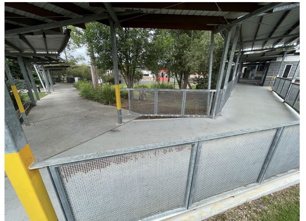
Photo 12: Overview of the pathed area within the northeastern portion of the site. Looking southwest.
