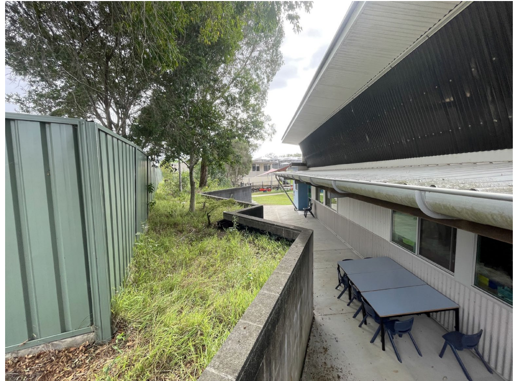
Photo 8: Overview of the western portion of the investigation area adjacent to the primary school buildings present. Looking north.
