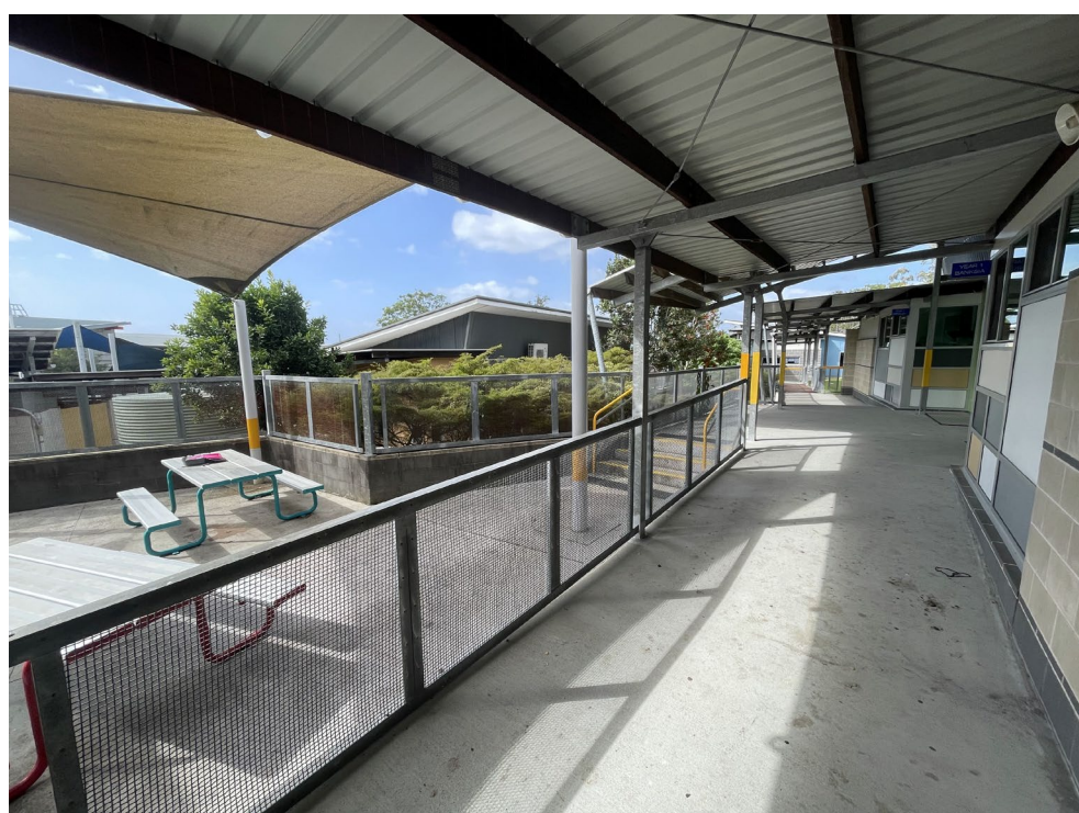
Photo 3: Overview of the Central portion of the investigation area, amongst the current primary school buildings present and in use. Looking south.
