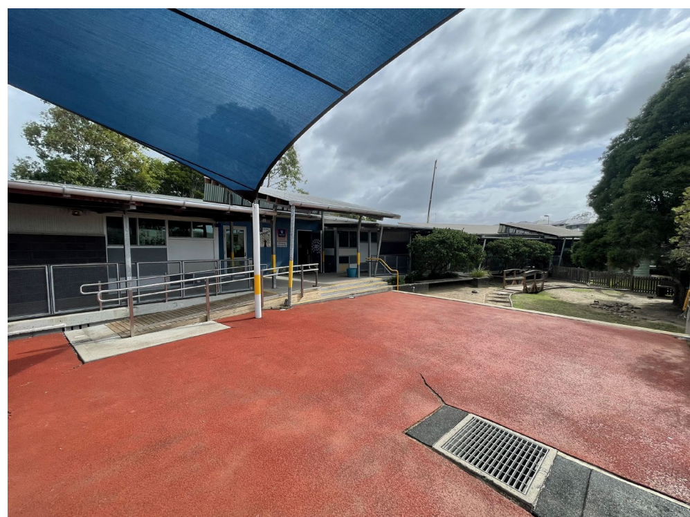
Photo 4: Overview of the central portion of the investigation area, amongst the current primary school buildings still in use. Looking north.
