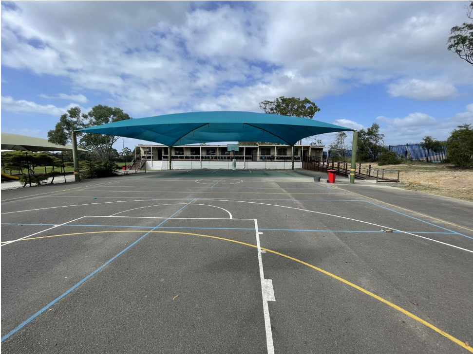
Photo 7: Overview of the basketball court within the southwestern portion of the investigation area. Looking south.
