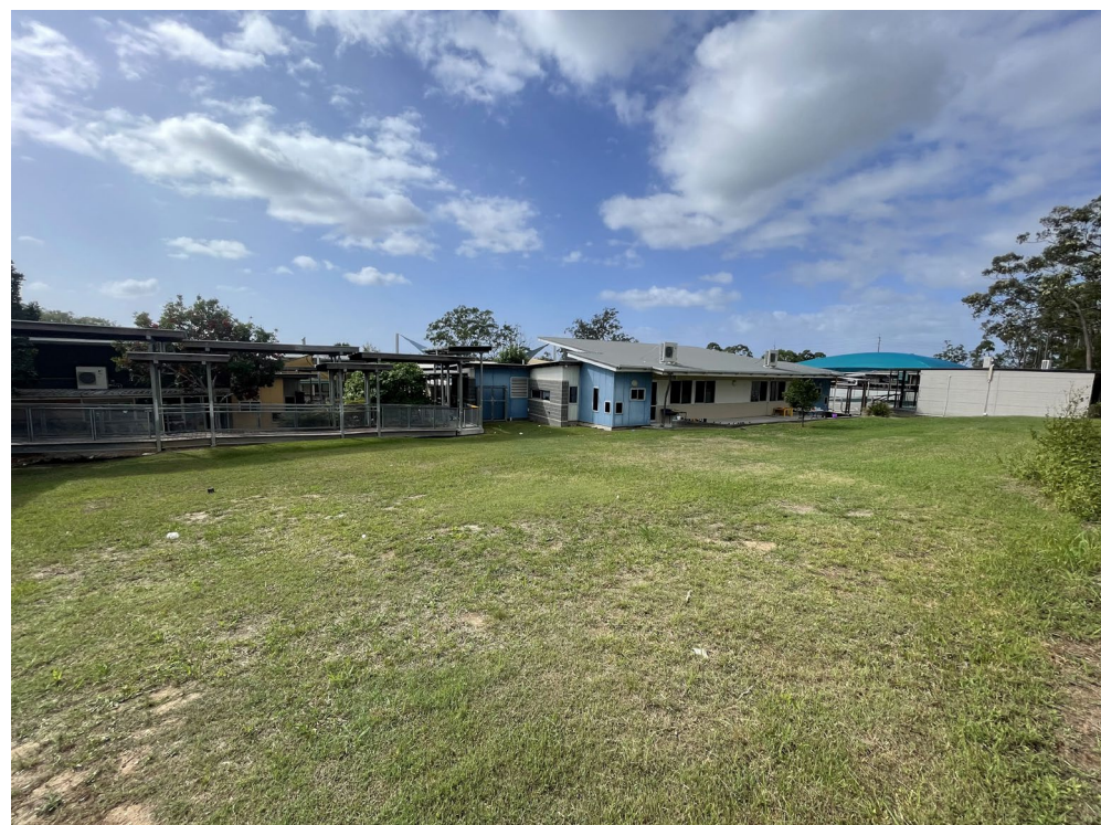
Photo 2: Overview of the central western portion of the investigation area, looking south.
