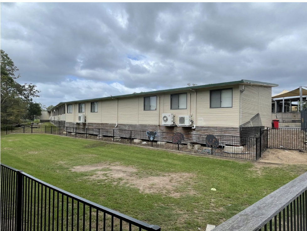
Photo 11: Overview of the eastern portion of the site and the primary school buildings present. The damaged boardwalk structure is present in the distance. Looking southwest.
